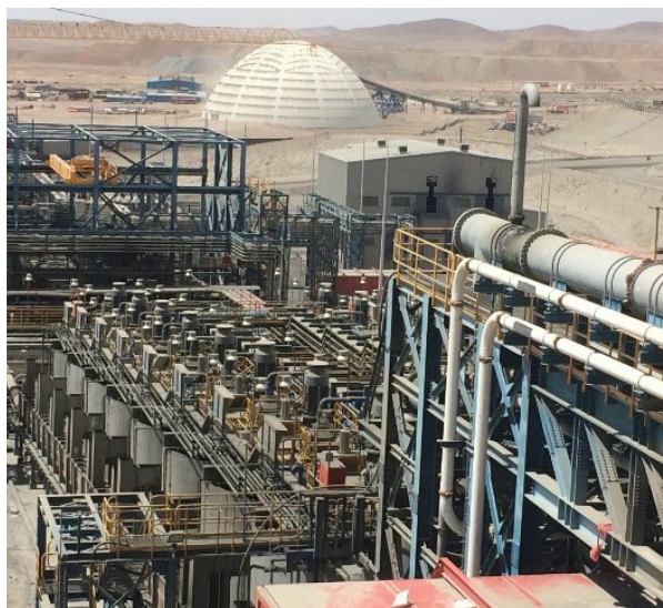
Flotation cells used in a preliminary stage of copper production in Chile.
